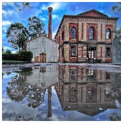
5. Walka Pump House
